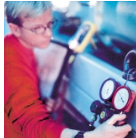
Accreditation is required for inspection of refrigeration equipment. This is essential in order to ensure safety and to protect the environment.
